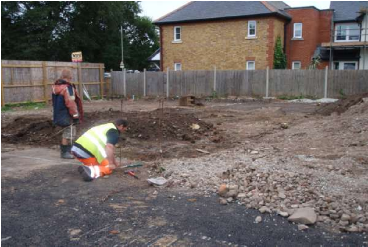
Plate 2. General view of site with setting out of trenches
