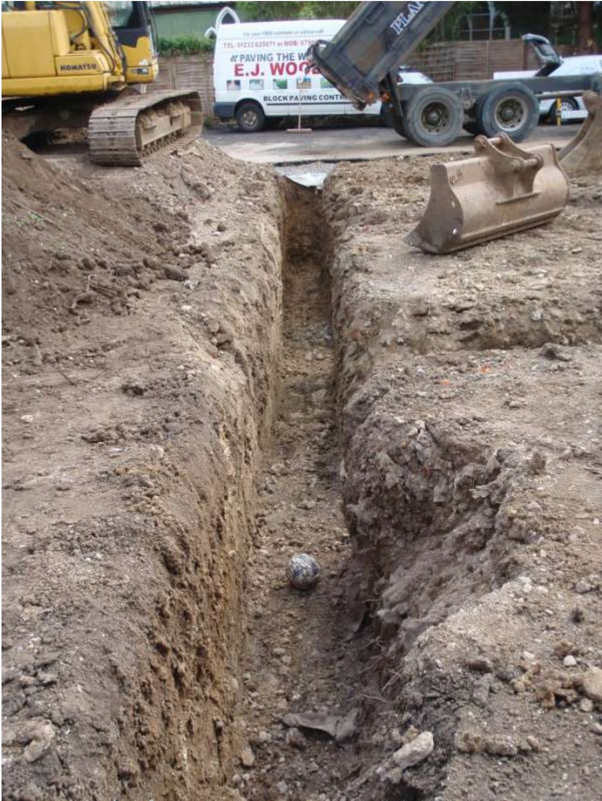
Plate 6. View of foundation trenches on the east side of the site
