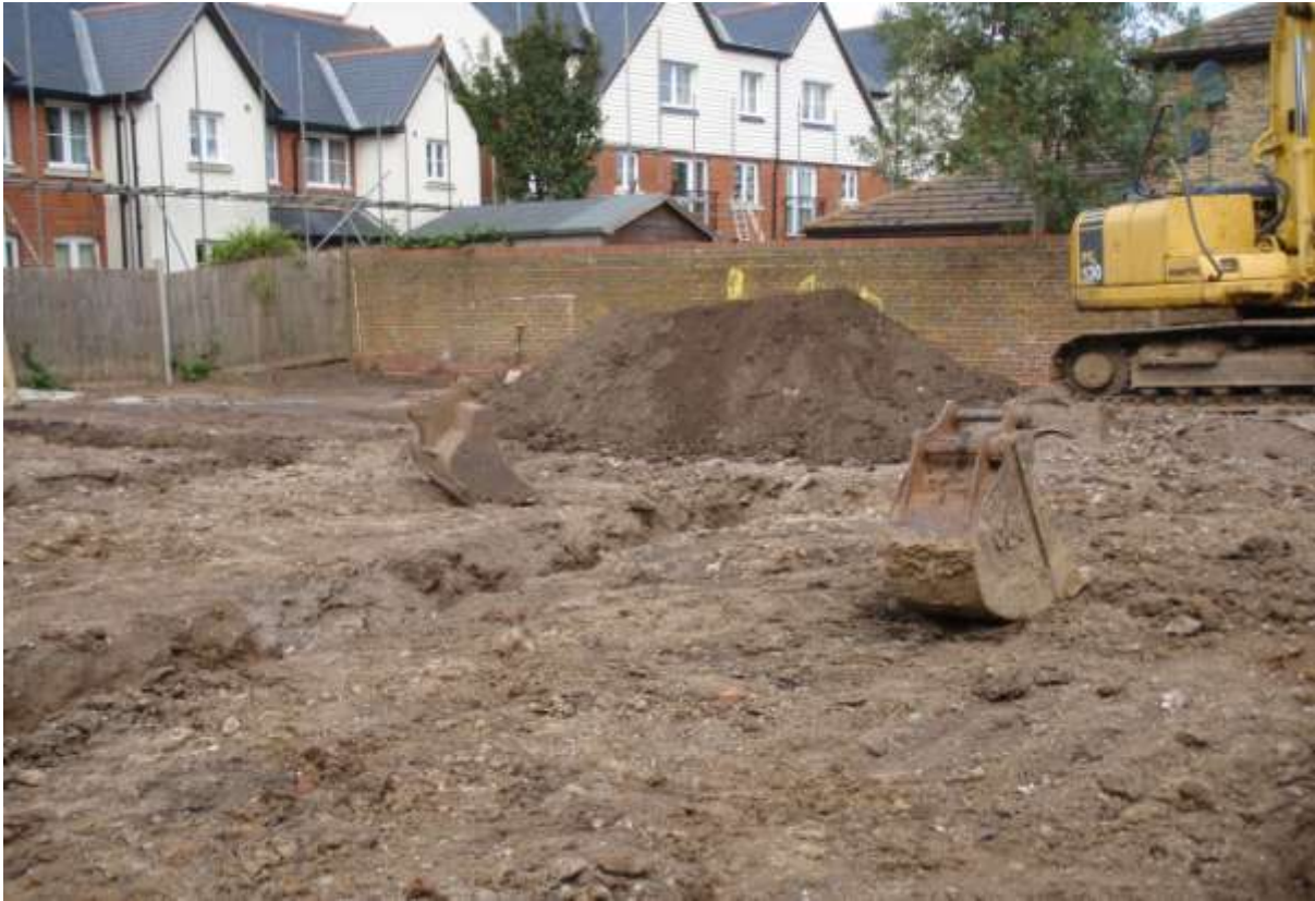
Plate 4. Foundation trenches on the east side
