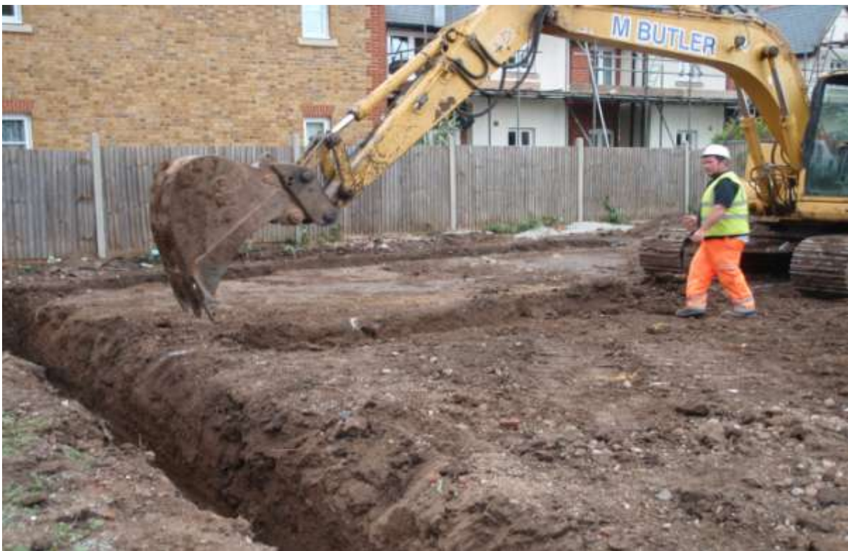
Plate 3. The site showing cutting of foundation trenches on the west side
